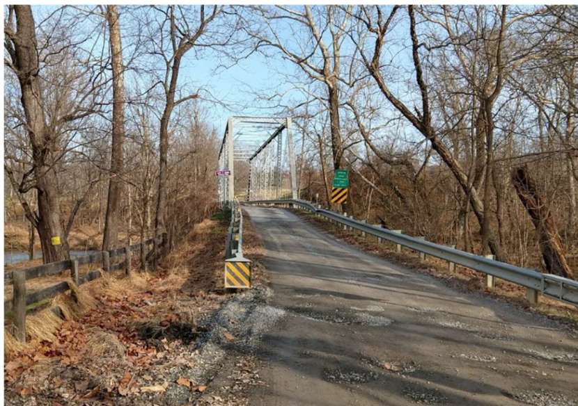
John G. Lewis Memorial Bridge over Catoctin Creek
