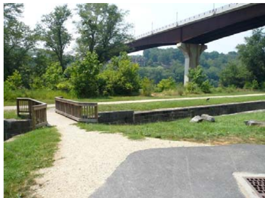
Start: Facing East
